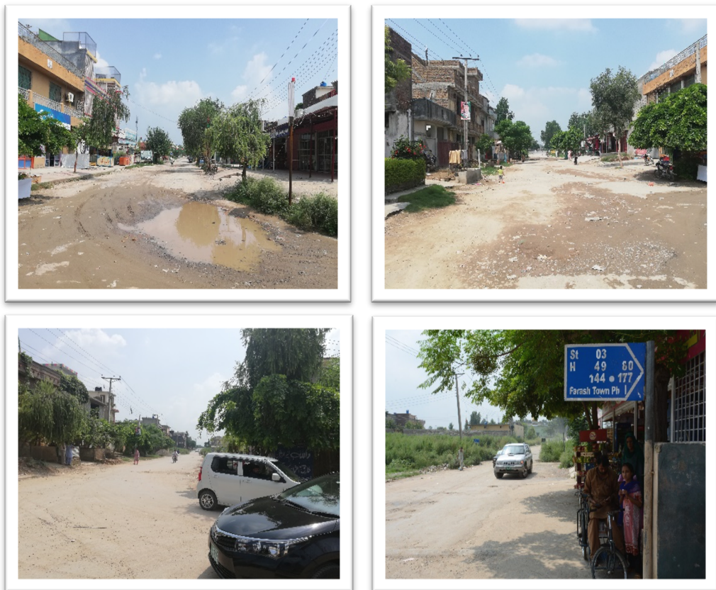
Figure 14-17. A view of Model Urban Shelter Project, Farash
